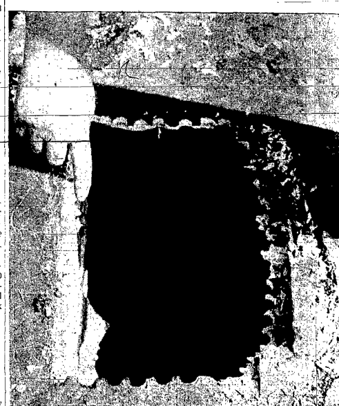
THIEVES WEDNESDAY morning drilled this 10-in. x 16-in. hole in the roof of Griess Rexall store to gain entrance. The hole is that of Police Chief R. H. Hansen and points to the jagged edges left by the drill.
